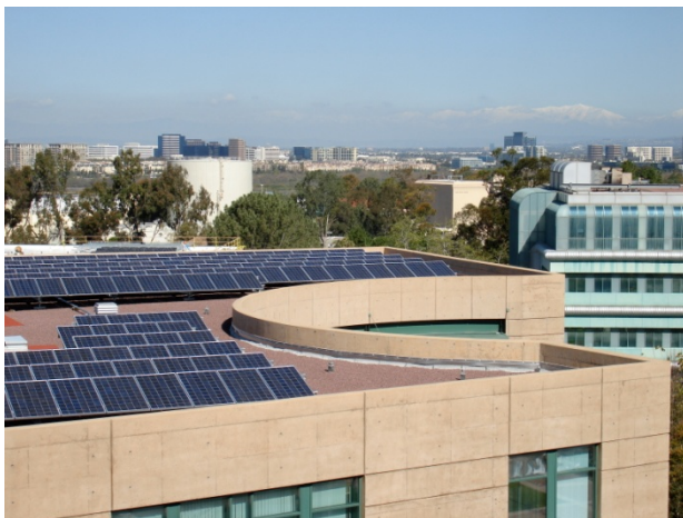
Solar panels on a UC Irvine roof
