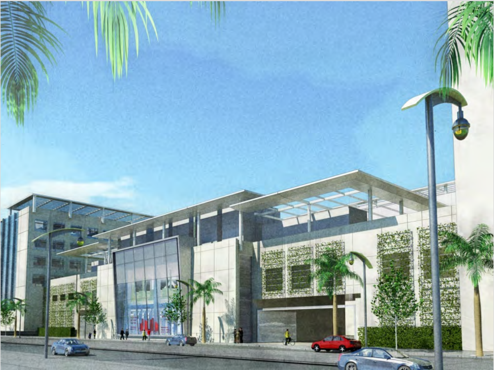
The Energy Center (East Side) 20
