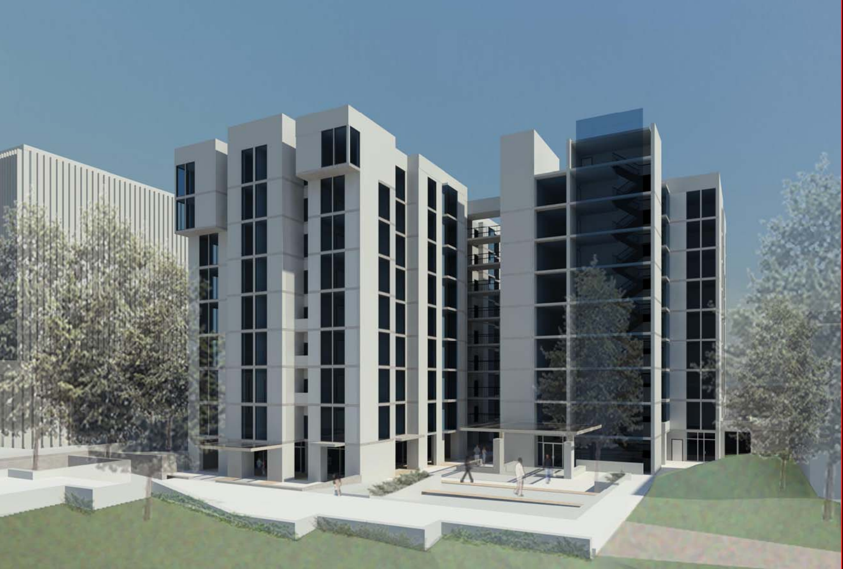
3-Dimensional Building View – View from Stewart Commons
