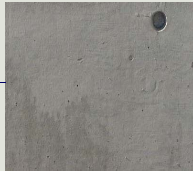
Concrete, architectural finish
