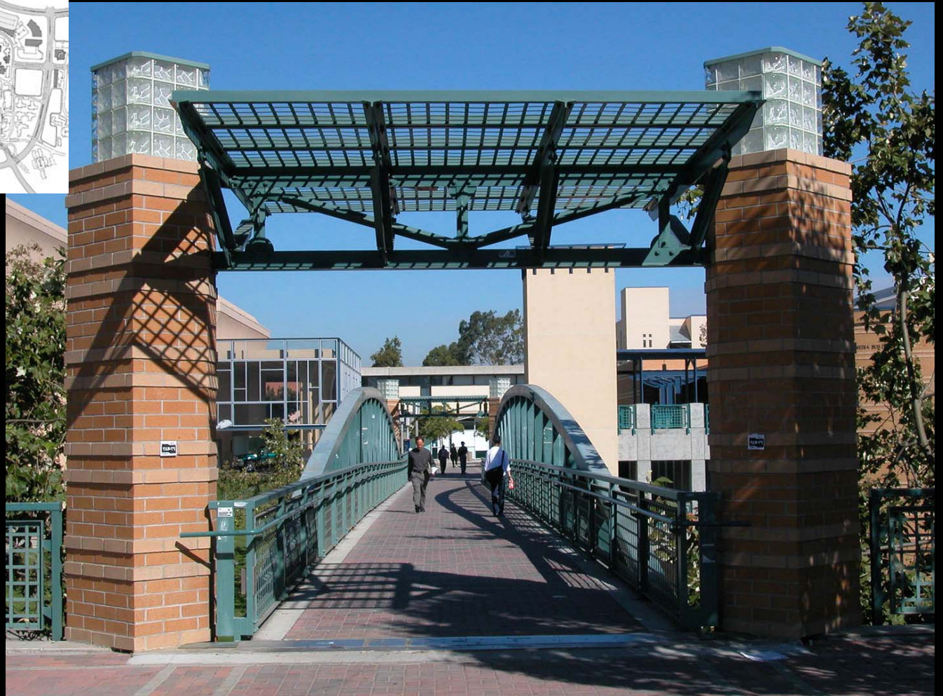
HUMANITIES/ARTS PEDESTRIAN BRIDGE
