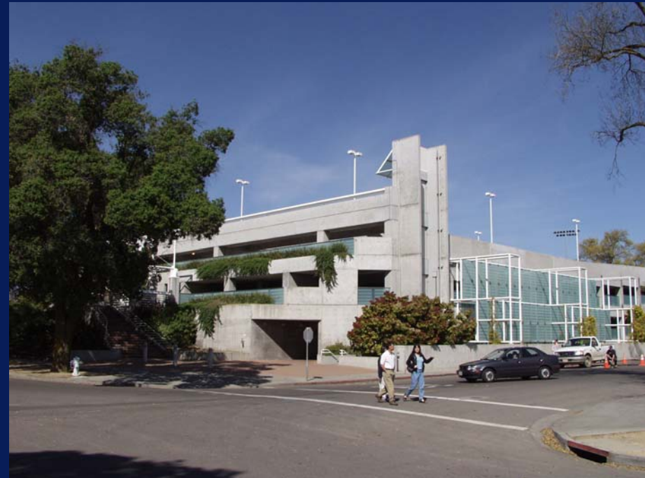
Howard Way Parking Structure
