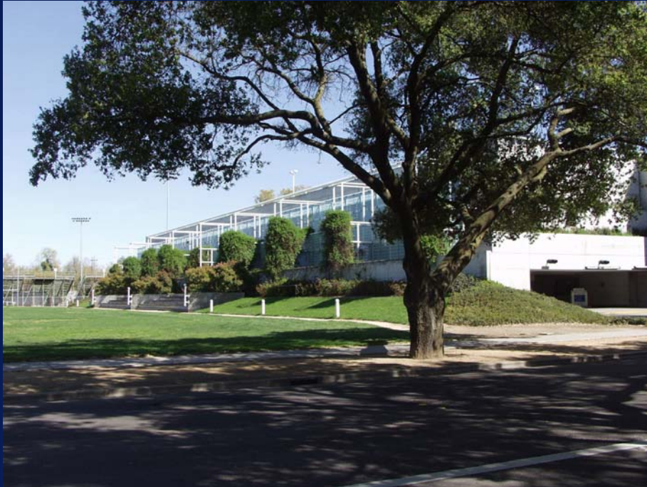
Howard Way Parking Structure
