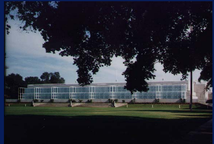
Howard Way Parking Structure
