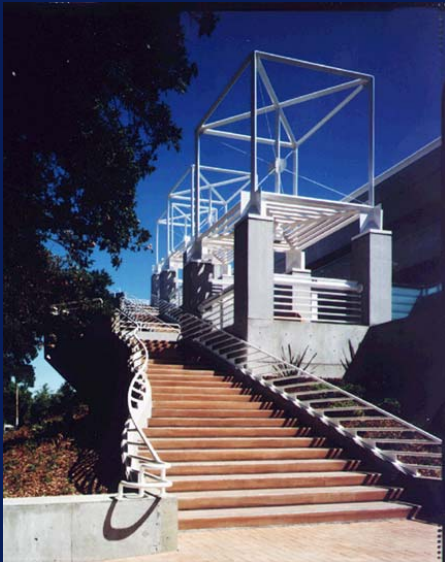
Howard Way Parking Structure
