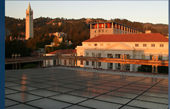
UC Berkeley's 100 kW PV array, located on Martin Luther King Student Center roof
