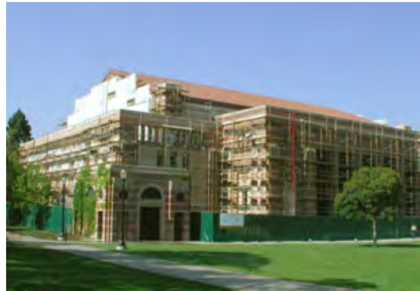
Student Activity Center Seismic Renovation (2004)
