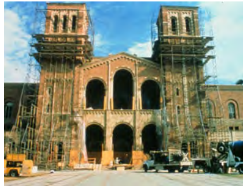
Royce Hall Seismic Renovation (1998)
