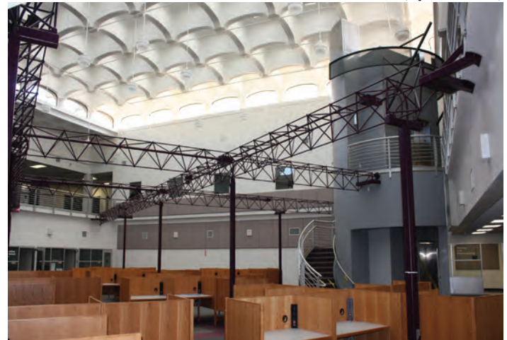
Galbraith Hall (before renovation)
