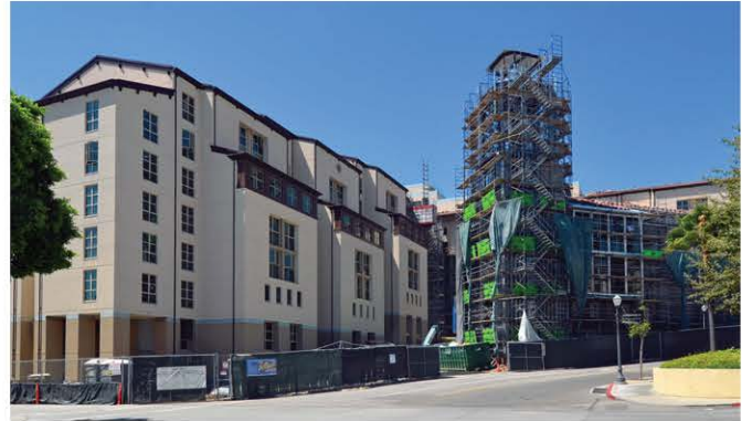
Weyburn Terrace Graduate Housing (in construction July 2012)
