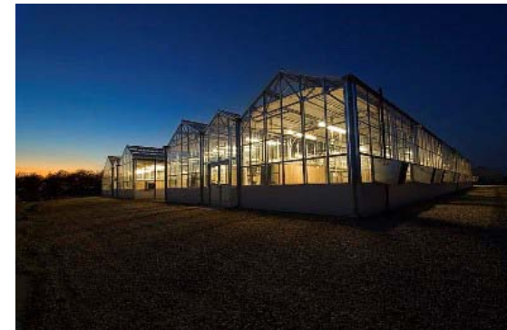
Kearney REC Greenhouse Facility
