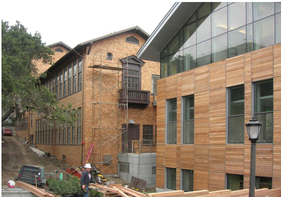
Blum Center Under Construction
