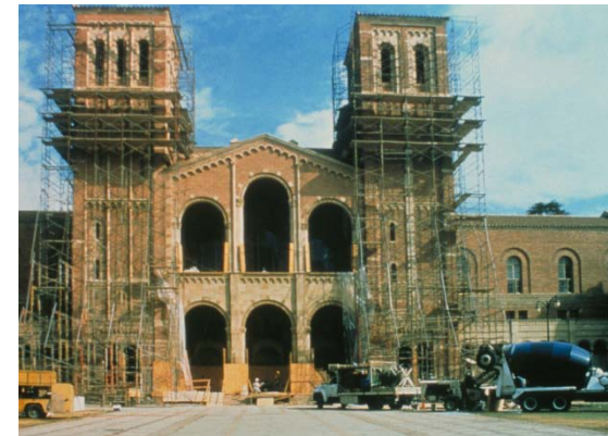
Royce Hall Seismic Renovation
