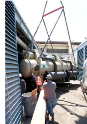
Installation of High-Efficiency Chiller
