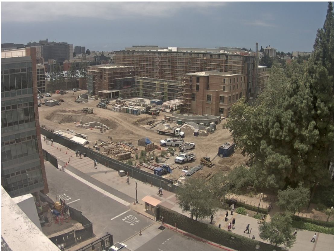
Under construction: Luskin Conference Center, UCLA
