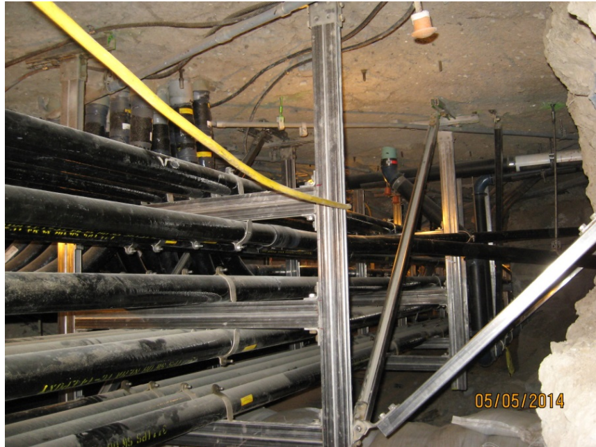
Rock Hall – below slab utilities replacement
