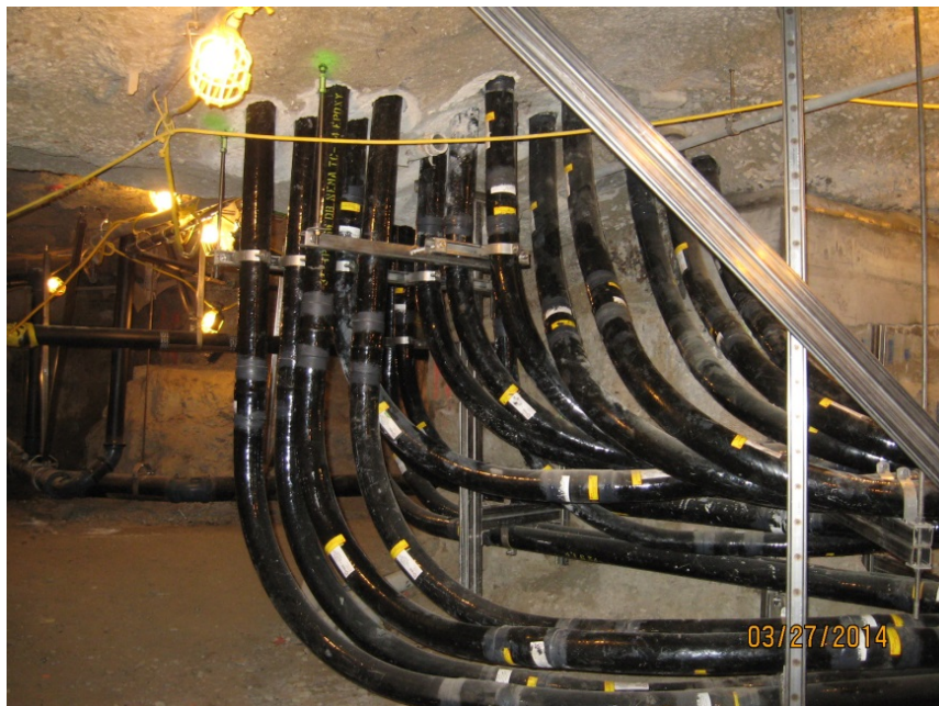
Rock Hall - below slab utilities
