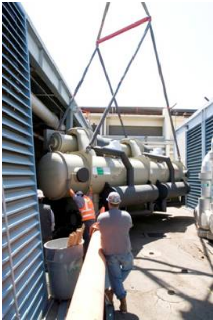
Installation of High-Efficiency Chiller
