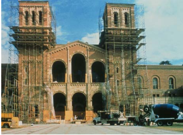
Royce Hall Seismic Renovations (1998)
