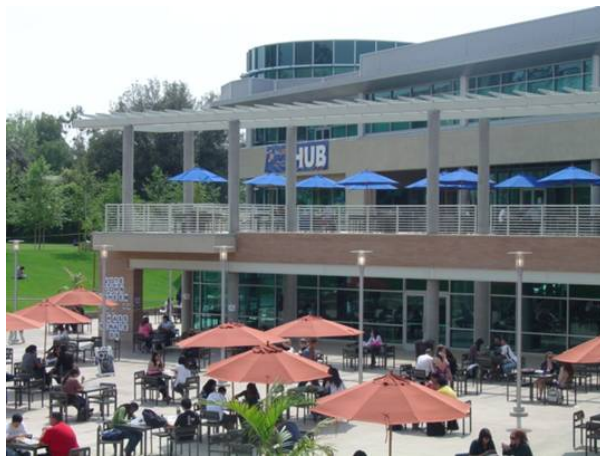
Highlander Union Building
