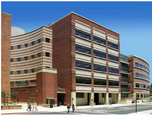
Biomedical Sciences Research Building (seismic replacement building) and Orthopedic Hospital Research Center
